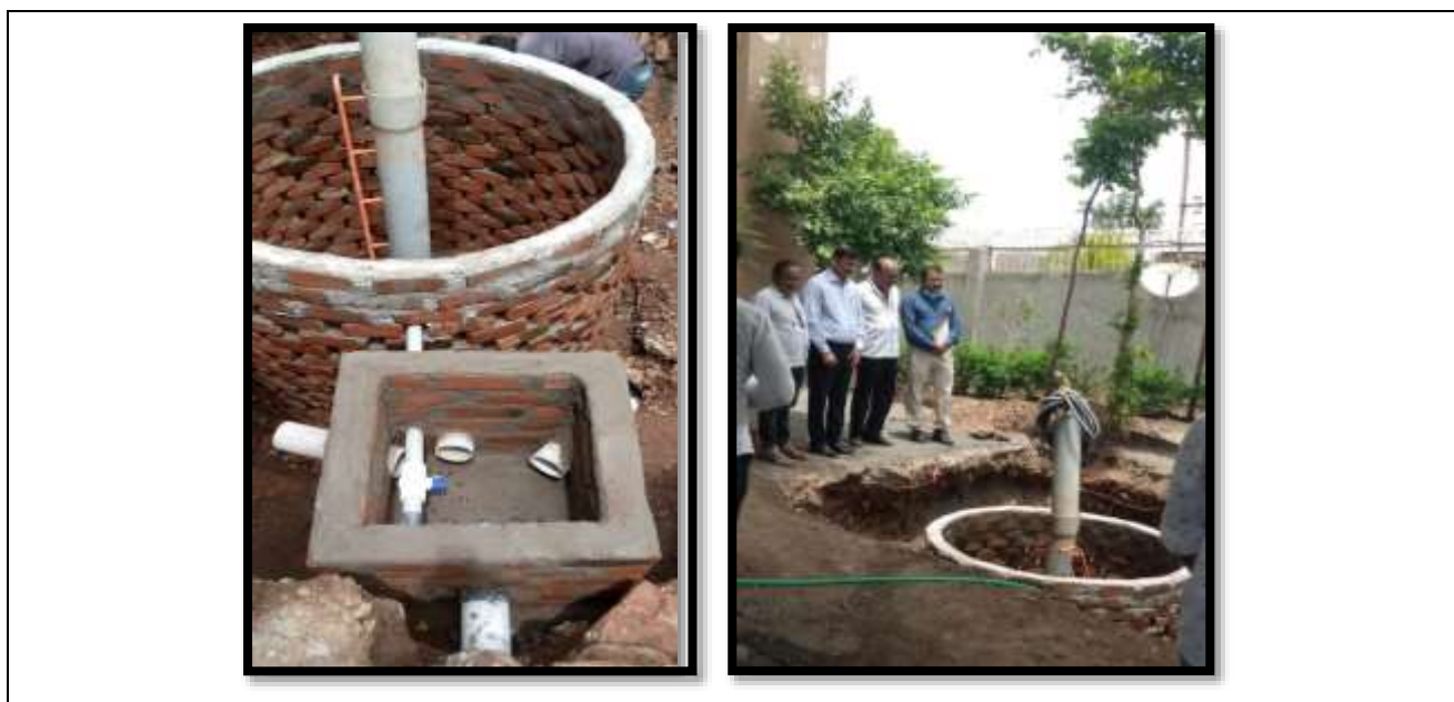
Rain Water Storage Well
